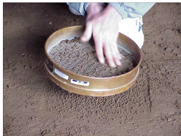
Filling surface voids
