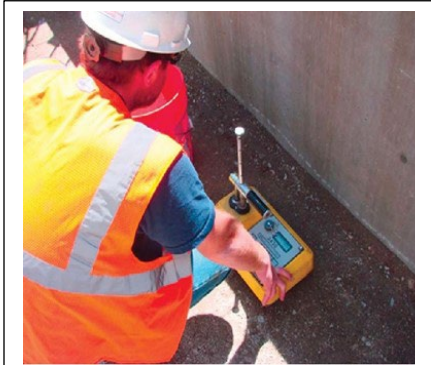
Testing near structure
