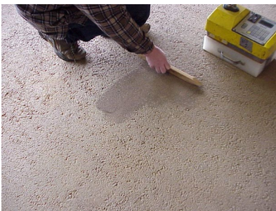
Filler on pavement
