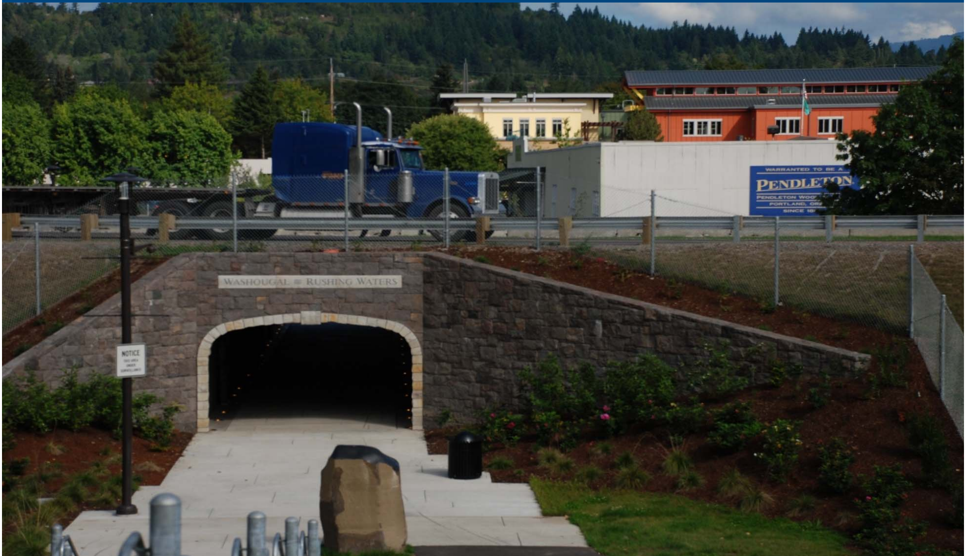
SR 14 Tunnel Washougal, WA
