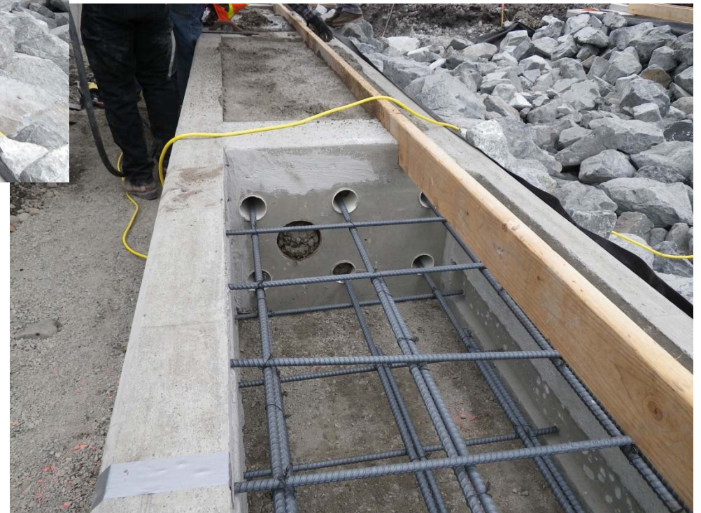
Madigan Bypass Realignment – Murray Creek Culvert Replacement JBLM, WA
