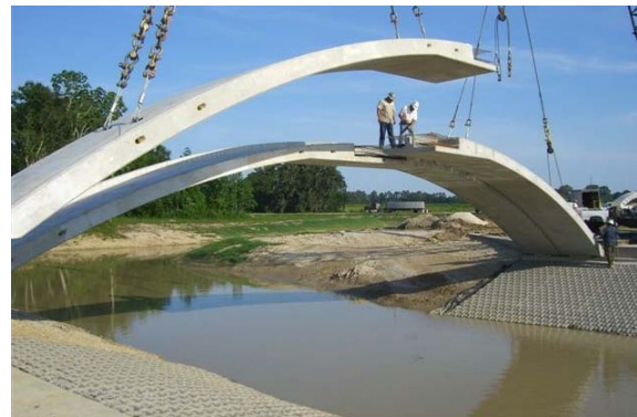
TWIN LEAF CONSTRUCTION
