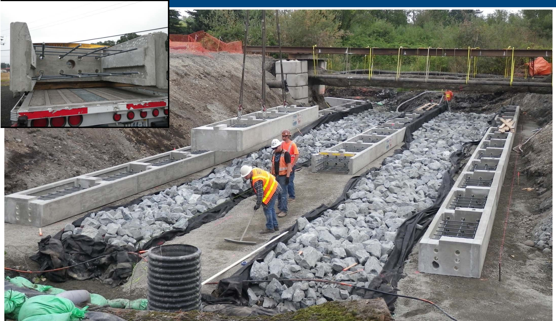
Madigan Bypass Realignment – Murray Creek Culvert Replacement JBLM, WA
