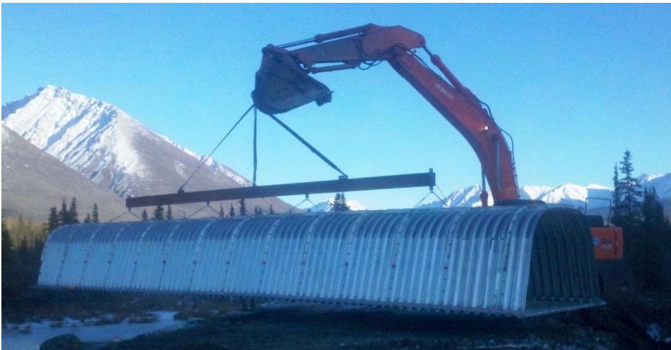
Chokosna Pond Culvert, McCarthy, AK
