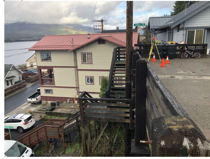
LOOKING N, STAIRCASE FROM SAYLES ST. TO WATER ST.
