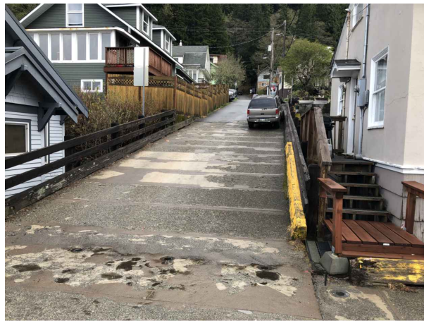
LOOKING NE, DOWNSTATION, GORGE ST.
