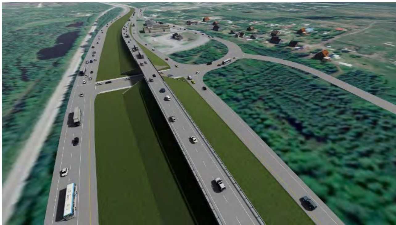
View from the West
