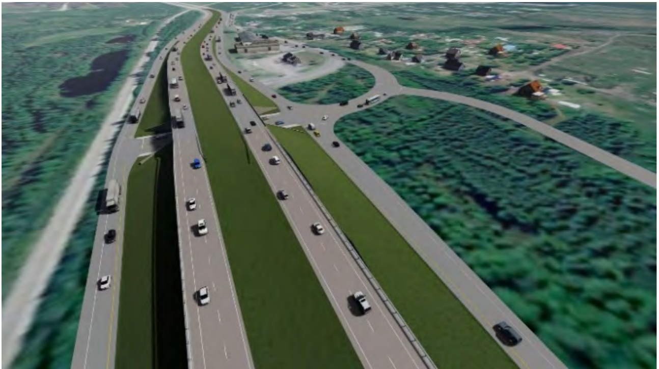
View from the West
