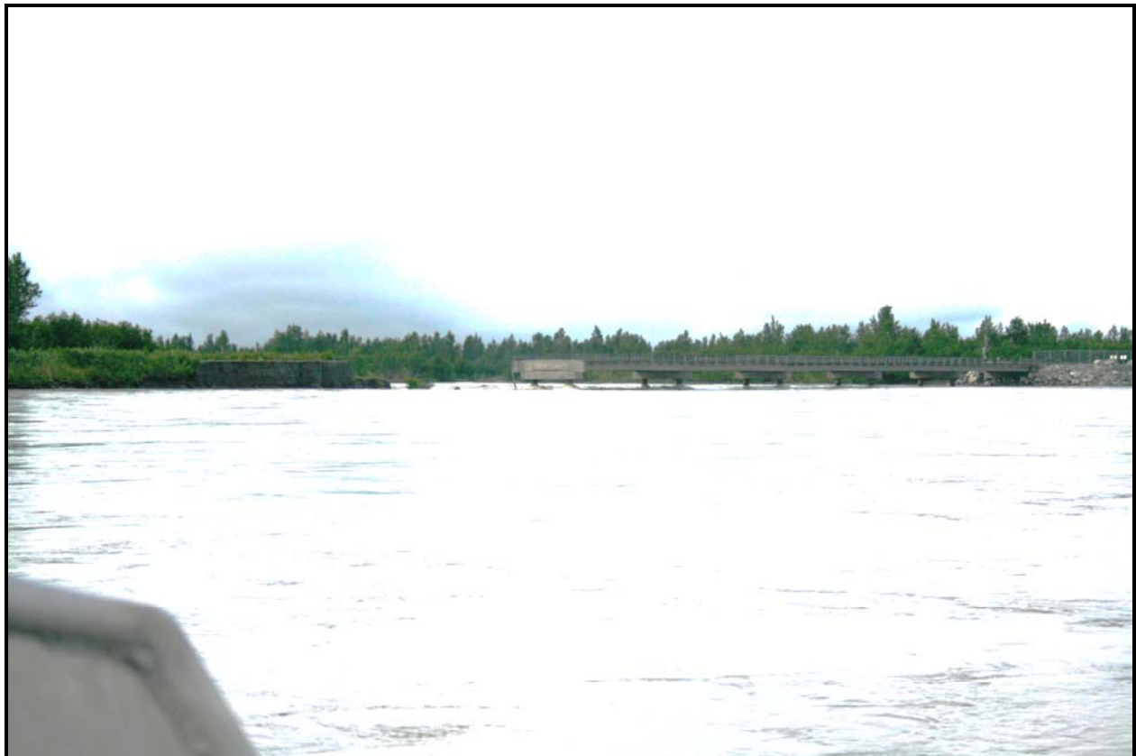
Figure 1 – Bridge 339 looking south August 14, 2012
